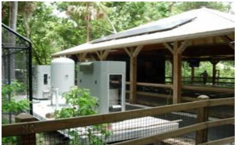
A 5 kW photovoltaic array on the roof of this pavilion runs an electrolyzer that generates hydrogen fuel for a Hydrogenics PEM fuel cell at Homosassa Wildlife Park, Homosassa, Florida.
