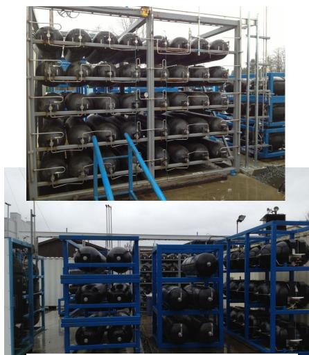
Examples of hydrogen storage (up to 950 bar) at Powertech
