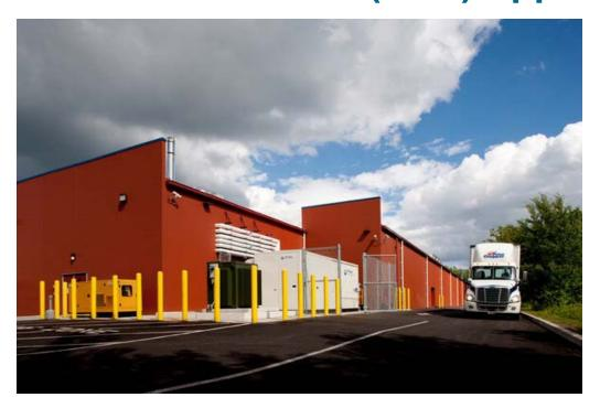
A 400-kW fuel cell (grey box) meets 85 percent of the energy needs of this Price Chopper supermarket in Albany. The installation reduces the building's carbon footprint by 71 tons, provides energy security for perishable items, and saves more than 4 million gallons of water each year. (Photo taken from the Executive Summary of the New York State Climate Action Plan Interim Report)
