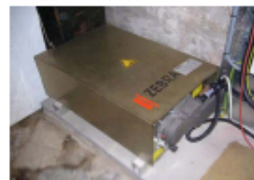
NiNaCl battery (Zebra, 2kW)
