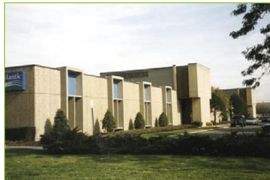
Figure 1. Verizon’s Garden City “central office of the future” gets most of its power, cooling, and heating from onsite engines and fuel cells, absorption chillers, and a HRSG.
