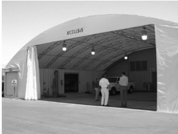
Figure 6. Outside of existing maintenance facility for hydrogen buses.
