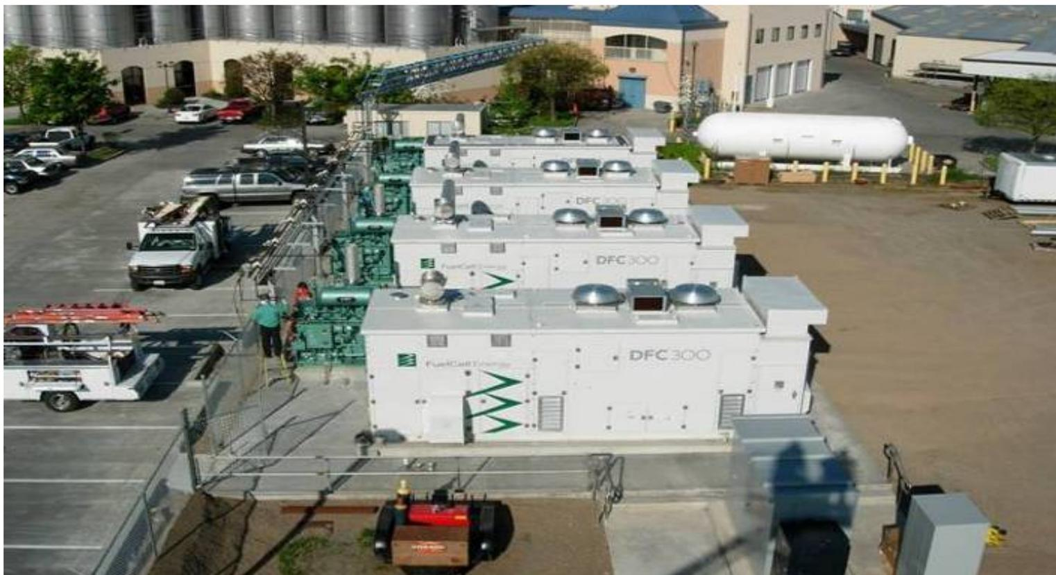
DFC 300 CHP, 1MW, digester biofuel and natural gas
