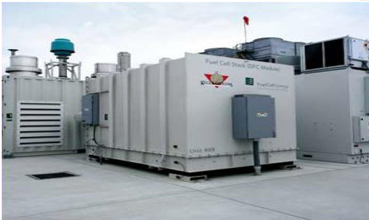
600 KW DFC 300 Units, digester fuel, combined heat and power
