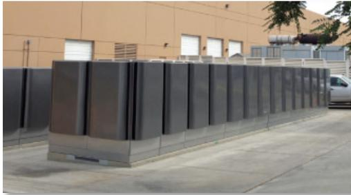
debuted its Bloom Energy fuel cell system that generates about 60% of the power needed for its Carlsbad, California headquarters and the manufacturing and distribution center. The new fuel cell system fits within 1,500 square feet and provides 1 MW of power that is generated onsite.
