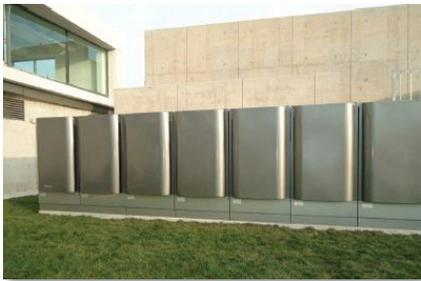
In April 2012, WGL Holdings announced a 200-kW natural gas-powered Bloom Energy SOFC had been installed at the new, LEED certified Washington Gas Springfield Center. The fuel cell runs round-the-clock and meets approximately 35% of the site's baseload power needs. By using the fuel cell, CO<sub>2</sub> will be reduced by approximately 50% compared to the grid.
