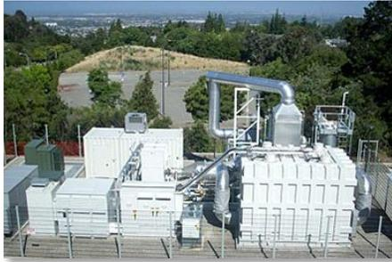
In June 2010, Pacific Gas and Electric Company (PG&E) ordered a 1.4 MW FuelCell Energy DFC1500 fuel cell power plant to install as utility-owned fuel cells at the campus of California State University East Bay – Hayward Hills (CSU – East Bay). Installed in 2012, the fuel cell power plant is configured to utilize the fuel cells' waste heat for heating a swimming pool and utilize the waste water for landscape irrigation.
