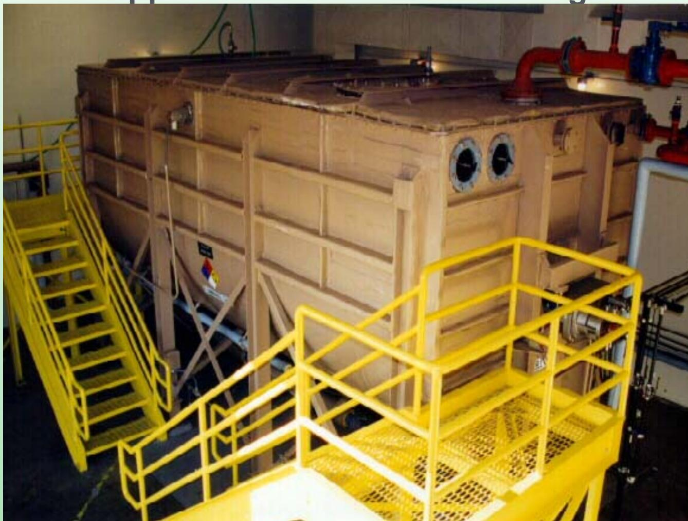
Photo of Plug Flow MSW Digester Courtesy of Pinnacle Biotechnologies
