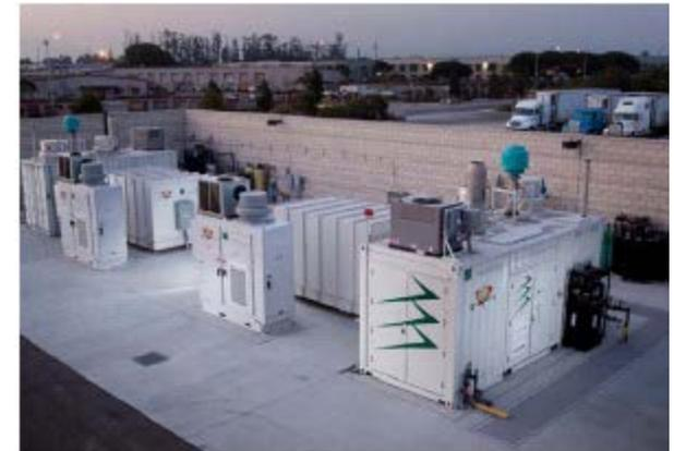
Digester processes 30,000 gal of onion juice per day, Producing biogas containing 70% methane
