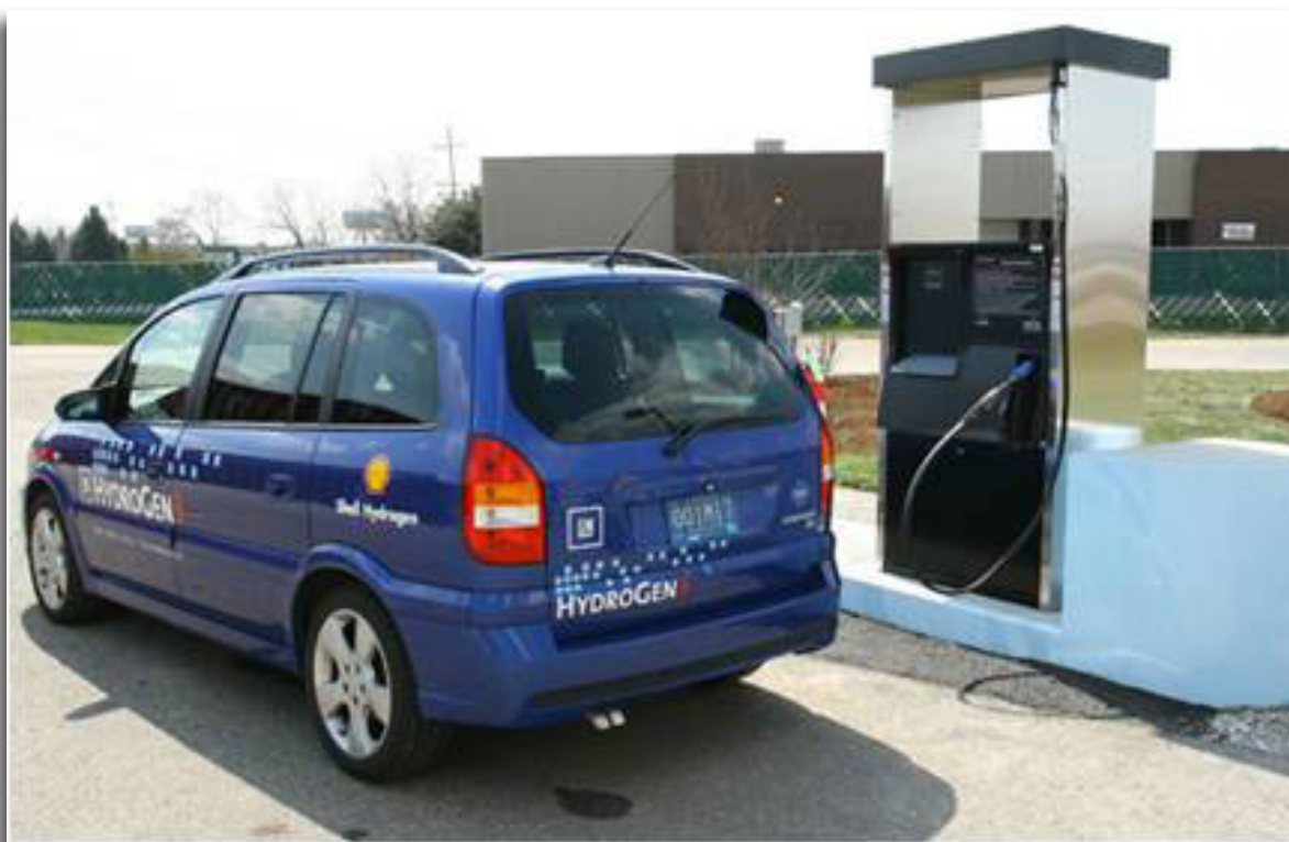
H2 ProGen Hydrogen Dispensing Station
