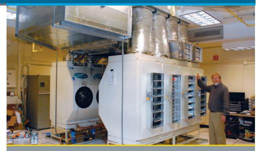
The above photo shows the multi-stage indirect evaporative cooling units installed at the National Snow and Ice Data center in May 2011. Photo used with permission from the National Snow and Ice Data Center.
