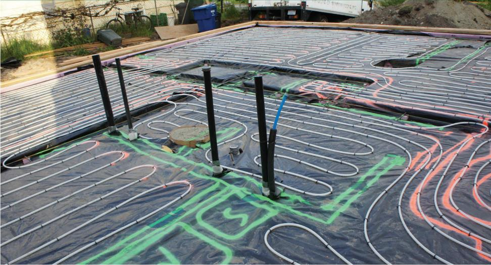
An air-to-water heat pump heats water for the radiant floor heating embedded in the first-floor slab. The concrete slab was stained to provide the finished floor surface. The home's south-facing windows allow in winter sunlight to warm the slab for passive solar heating.
