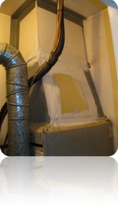
• *Rigid trunk duct* and *trunk to flex duct connections* in the attic with mastic – where accessible
