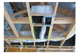
Insulated attic coffers were utilized in key locations to allow for the placement of ductwork in conditioned space without dropping the ceiling. This maintained the indoor aesthetic in rooms such as kitchens, living and dining areas, and wide open spaces.
