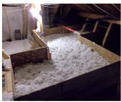
Mechanical closet in attic (left photo) and insulation "trough" installed over ceiling coffer (right photo) to ensure consistent levels of ceiling insulation over duct coffers
