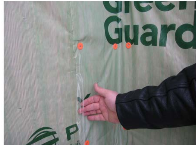
Figure 1 - The tape shown here was not firmly bonded to the house wrap.
