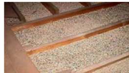
Vermiculite insulation between attic joists (image courtesy of EPA ).
