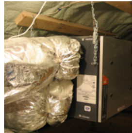
This HRV, installed in a con provides balanced ventilati home
