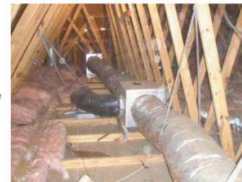
A ducted central return brings air from central return registers back to the air handler through insulated, air-sealed ducts
