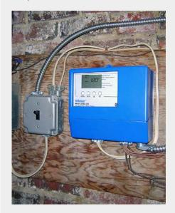
In the three buildings, new boiler control systems were installed and achieved 10%–34% energy savings.
