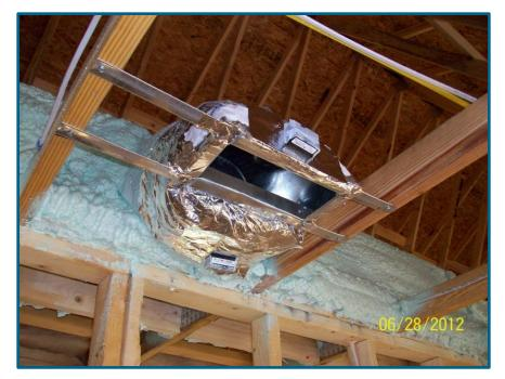
**Approach**: Work with a production builder to develop optimized compact buried duct designs and monitor in-service performance
