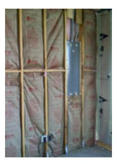
Inset stapling was used to fasten the insulation to the sides of framing, which created a thermal bypass. The builder restapled the kraft tabs to the stud faces to remedy this problem.
