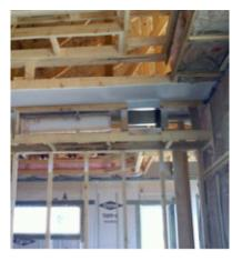
After the ceiling drywall was installed, the ducts were installed in chases beneath the ceiling providing a conditioned space for the HVAC ducts with a continuous air barrier above.
