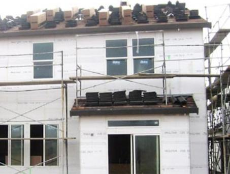
Taped rigid foam insulation can serve as a drainage plane and air barrier as well as a thermal boundary behind a stucco cladding. If using housewrap instead, never apply stucco directly to plastic housewrap. Provide a drainage space to prevent wetting of the housewrap or use two layers of textured building paper.
