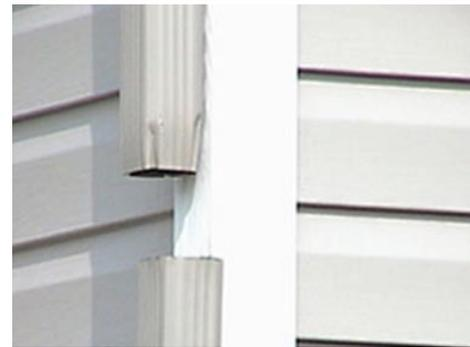
Install flashing at roof valleys and edges and install rain gutters to guide water off roof and away from house. Make sure the downspouts are connected and extend to at least 3 feet from the house. (Photo source: EPA, photo by Terry Brennan)
