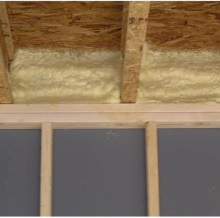
Sealing gaps between floor joists with spray foam provides a good air seal that prevents the flow of heat, cold, and pollutants from unconditioned space to conditioned space.
