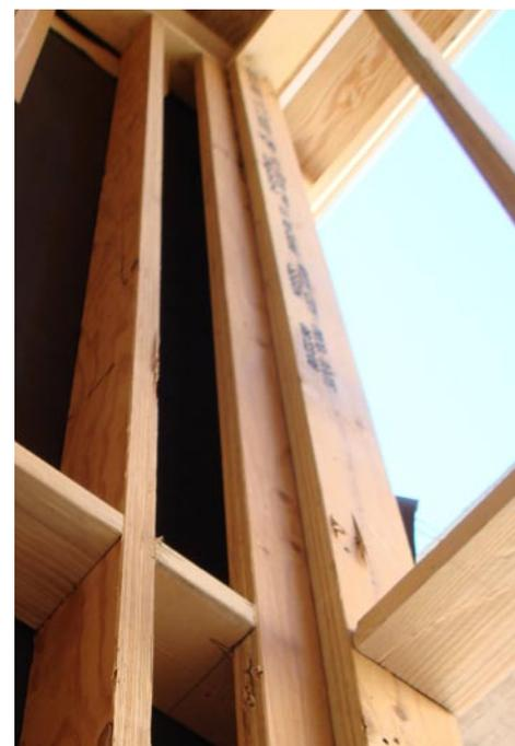
Using dry wall clips or a 1x nailer strip to avoid the third stud in corners provides more room for insulation and reduces lumber.
