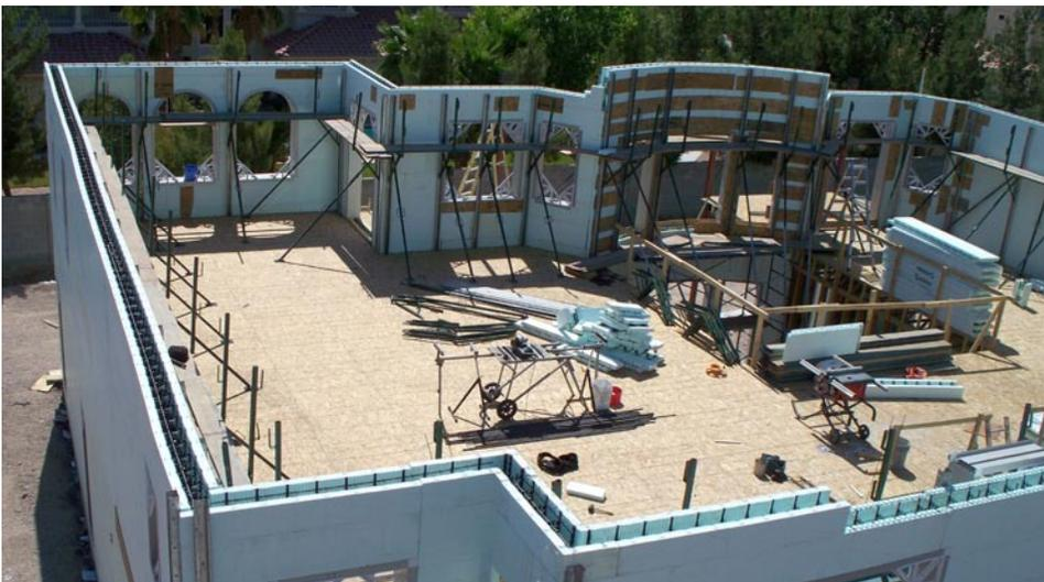
Insulated concrete form (ICF) walls form a solid thermal boundary for the NextGen 2009 home in Las Vegas.
