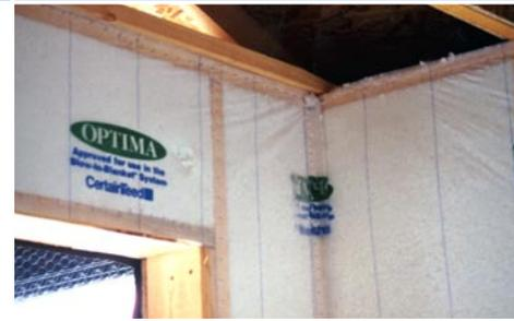
Centex of Northern California used a system it calls “zero defect” wall insulation in homes in San Ramon to help achieve energy savings of almost 40% over the Building America benchmark. It includes 2x6 framing to accommodate R-23 blown fiberglass in walls for more consistent fill than fiberglass batts, R-38 in the ceiling to cover ducts, and careful caulking and sealing of all joints and penetrations to reduce air leakage.
