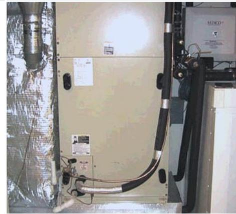
The first-generation zero-energy home contains an AC unit and an integrated solar water and space heating system. In the second-generation home, solar collectors provide water heating with backup water heating provided by a tankless gas water heater and space heat provided by an air source heat pump (Photo source: by NAHBRC).
