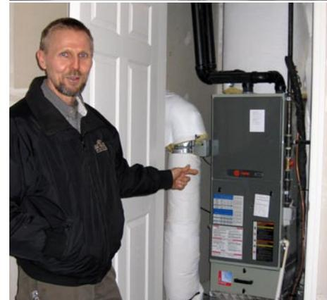
This builder points to a mechanized damper on a fresh air intake to the HVAC air handler. The damper can be set by a timer (shown above) to open allowing fresh air to be pulled into the air handler by the fan, also operated by the timer. This draws fresh air into the house at regular intervals.
