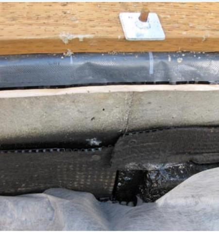
This foundation moisture management approach uses a dimpled-plastic drainage plane and damp proofing on the exterior side of the foundation wall. Landscape filter fabric keeps soil from clogging the gravel around the perforated drainage pipe. A gasket keeps moisture from migrating up through the footing into the treated sill plate.
