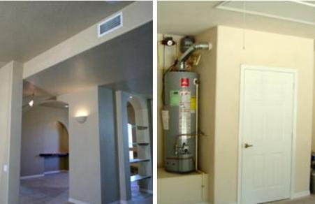
(top) One technique for placing ducts in conditioned space is to run a duct chase in a dropped ceiling down the main hallway of the house with registers off the sides for each room. This technique allows for compact duct design.
