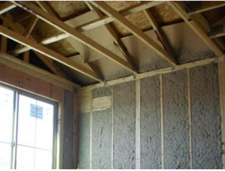
Baffles allow ventilation while keeping wind from blowing insulation back from the edges of an attic, when ceiling insulation is added.
