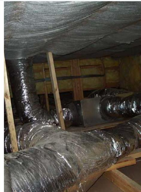
Ducts are located in conditioned space and mastic sealed to minimize heating and cooling losses.
