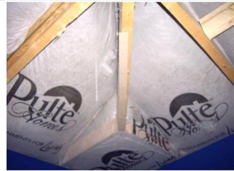
Pulte’s unique method of applying attic insulation keeps the blown cellulose right up against the roof line. This insulated attic provides conditioned space at the air handler and ducts at around 80°F instead of the 150°F temperatures found in uninsulated Las Vegas attics.
