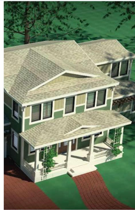
Light-colored roofing, like the roofing specified for the Environments for Living demonstration house at the 2009 International Builder Show in Las Vegas, can help minimize heat gain from solar radiation. Reflective roofs help keep homes (and surrounding neighborhoods) cool and help offset carbon emissions.
