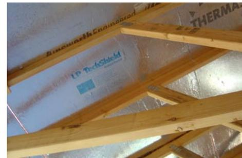
Radiant barriers can significantly reduce solar heat gain through the roof.
