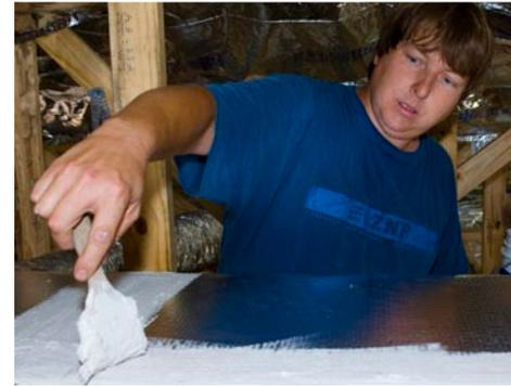
Mastic provides the most reliable duct sealing method. Ducts should be located in conditioned space. (Photo source: BAIHP)
