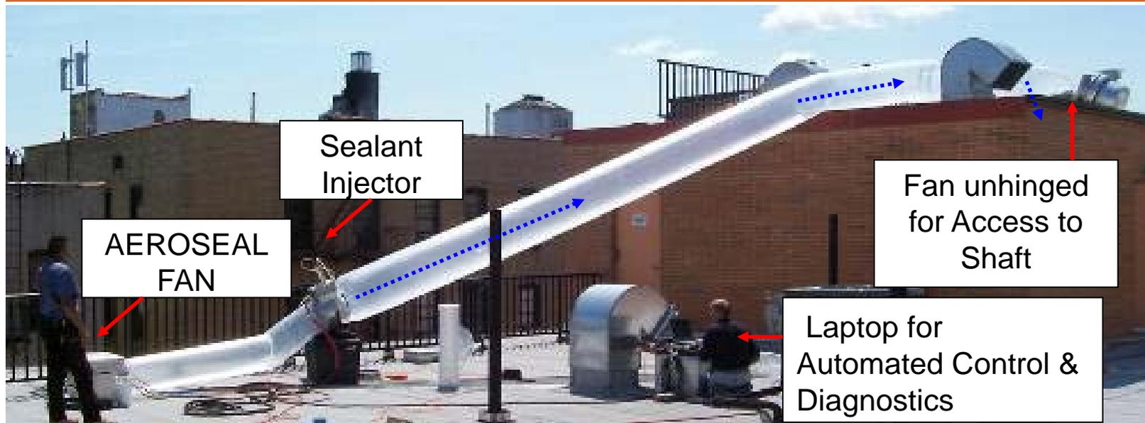
Aeroseal® aerosol duct sealant sticks to holes in ductwork and seals them
