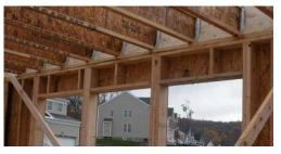
The rim joist for the second-story floor provides adequate structural strength so solid headers are not needed above first-story windows, allowing more room for insulation.
