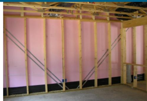
To save both money and energy, Urbane Homes used advanced 2x6 framing at 24-inch on-center, and sheathed exterior walls with XPS rigid foam instead of OSB.
