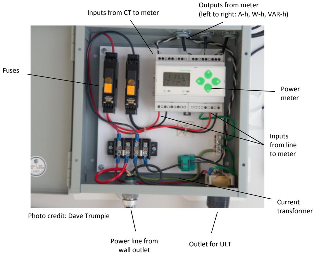
**Figure C.3: Photograph of Power Meter Inside Electrical Box**
