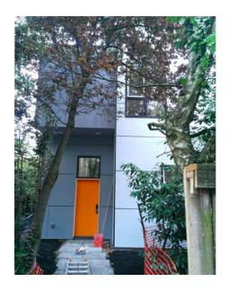
Long-lasting fiber cement siding and standing seam metal roofing provide durable exterior finishes in the often damp Northwest climate.
