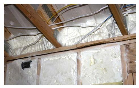
Closed-cell spray foam was used judiciously to seal and insulate above the top plates on all interior and exterior walls. Closed-cell spray foam was also used to air seal and insulate all of the rim and band joists.
