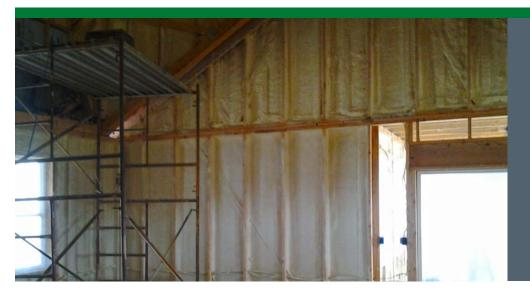
The builder used a "flash and batt" approach to wall insulation consisting of spray foaming the cavities with 1.5 inches of closed-cell spray foam, then filling the remainder of the walls with blown fiberglass. A coated 1-inch-thick rigid foam EPS sheathing was used on the exterior of the walls. The seams were taped with polybutyl tape to form a weather-proof air barrier under the resinand-wood composite siding.
