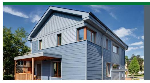
The home meets the Passive House Institute's strict criteria for air tightness and insulation. The builder employed several types of insulation and flashing in the 19-inch-thick walls and roof to provide redundant layers of protection against the elements.
