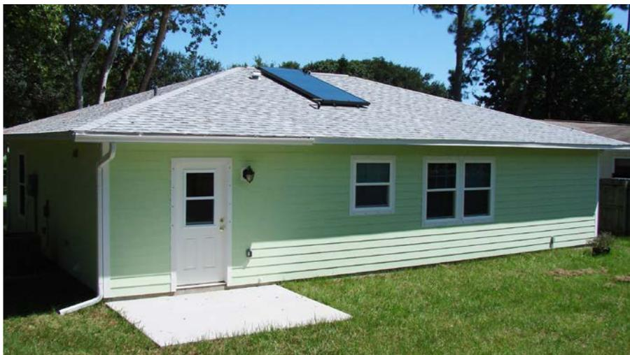
Solar thermal panels, mounted on the south-facing rear roof, provide plenty of hot water at a cost of only \$121 a year to run, compared to \$282 a year for a conventional, 89%-efficient water heater.
