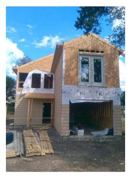
Textured house wrap provided a weatherresistant barrier over the SIPs and a drainage plane and slight air gap behind the vinyl siding.
