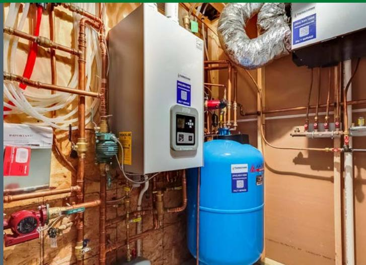
The home's heating, ventilating, and air-conditioning (HVAC) system is based on radiant in-floor heat with nine separate zones (which also provide thermal mass with tile for passive solar). It has a 110,000-Btu, 95% efficient boiler that provides domestic hot water and in-floor heat. A forced-air, 95% efficient, two-stage, fully modulating furnace on two electronic zones provides backup heat.
