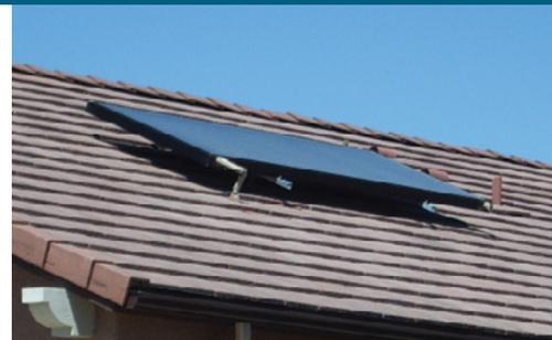
Solar water heaters generate 2,200 kWh/year, enough to recoup the cost of the system within 4 to 6 years.
