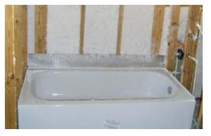
Tommy Williams Homes addresses common thermal bypass issues like heat loss around tubs and showers installed on exterior walls and at attic kneewalls by filling the wall cavities with blown fiberglass and covering them with a rigid air barrier material to prevent heat loss due to air flow.
