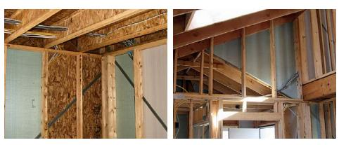
Advanced framing techniques such as two-stud corners and stacked framing (above left) save labor and materials, but they also simplify the installation of spray foam insulation and reduce the number of air leakage paths. However, complex framing to create architectural details (above right) needs to be considered carefully in order to ensure continuity of the air barrier system.
