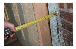
Closed-cell spray foam inside the brick walls provided excellent air sealing as well as insulation. With triple-pane windows and R-50+ roof insulation, the thermal loads on the apartments can easily be met with small heat pumps.
