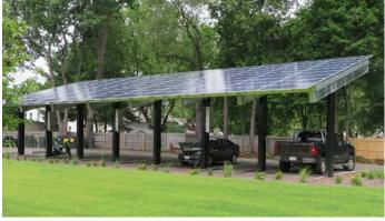
Roof space was not usable, so Olive Street Development chose to install the 30-kW PV system above the main parking area. Evacuated tube thermal collectors (for water heating) were installed as awnings over southern windows.
