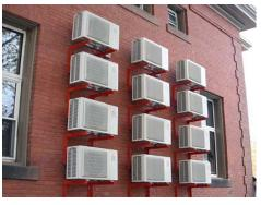
Ductless heat pumps provide most of the heating and cooling for the apartments. Finding room for all the outdoor units was a challenge; most were tucked on the rear wall of the building.
