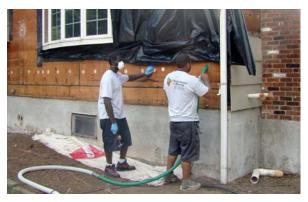
The siding replacement provided an opportunity to properly insulate the walls. A strip of sheathing was removed along the perimeter of the home to allow the old batt insulation to be removed. Once the sheathing was repaired, holes were drilled and cellulose was blown into the wall cavities. An infrared camera was used to verify that the walls were completely filled.
