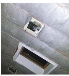
The vented attic over the bedrooms was converted to warm storage by applying closed-cell spray polyurethane foam (ccSPF) to the roof deck to make an unvented attic. In the cathedral ceilings, drywall was removed to allow for 3 in. of ccSPF to be applied to the roof deck before dense-packing the remaining roof rafters with cellulose.
