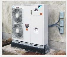
Chico Green Builders of Chico, CA, used the Altherma packaged AWHP product from Daikin. This high efficiency product provides hot and chilled water for space conditioning as well as domestic hot water.
