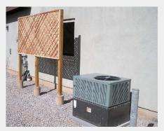
La Mirada Homes of Tucson, AZ, purchased a stand-alone refrigerant-to-water heat exchanger from AquaProducts, which packaged the heat exchanger (mounted underneath) with a standard heat pump. High efficiency heat pumps will increase system operational efficiencies.
