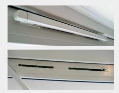
A typical trickle vent, shown installed in a window frame (top) and with the cover removed (bottom).
