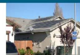
Premier Homes chose photovoltaic tiles that lie on the roof shingle-fashion and blend in with the concrete roofing tiles.
