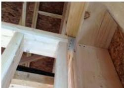
I hadn't seen this detail in the field before it showed up here, but I am pretty excited to see it now. Usually when we talk about interior walls intersecting with exterior walls in the context of energy-efficient framing, we talk about ladder backing as nailers rather than 3-stud wall bucks. And we talk about continuous sealant at the top and bottom plates and along the edges of the stud.
