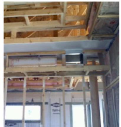
After the ceiling drywall was installed, the ducts were installed in chases beneath the ceiling providing a conditioned space for the HVAC ducts with a continuous air barrier above.
