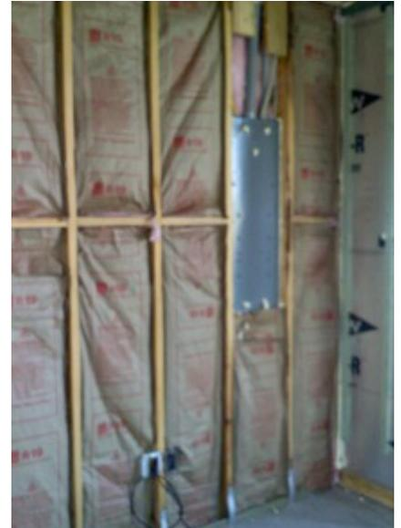
Inset stapling was used to fasten the insulation to the sides of framing, which created a thermal bypass. The builder restapled the kraft tabs to the stud faces to remedy this problem.
