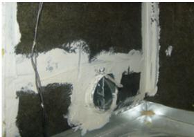
Typically air handlers are located in garages in Florida. (*Left*) In these homes the air handler was located in a closet inside the home to improve air quality and energy efficiency. (*Right*) A fresh air intake is ducted to the return air plenum to bring in fresh outside air that is filtered and tempered by the central air handler before being circulated throughout the home. (Photo Source: Florida Solar Energy Center)
