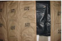
(left) In the crawlspace, R-30 fiberglass batts were installed between the 2x10 floor joists. The joists were then covered with 1 inch of expanded polystyrene (EPS) rigid foam board that was taped at the seams to provide a continuous air barrier and flashed at the edges to protect against rodents. The crawlspace floor was covered with a 6-mil visquene vapor barrier.
