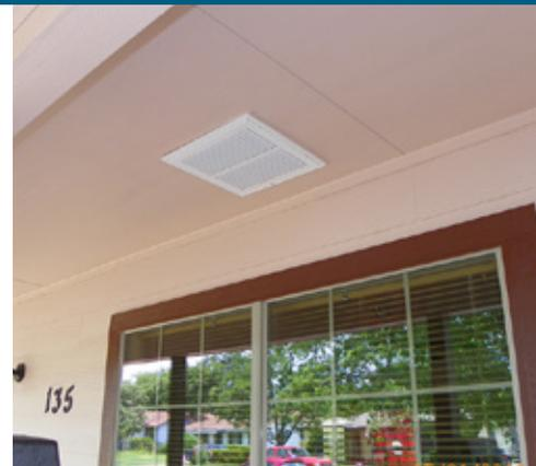
Transfer grilles (left photo) were installed to ensure good return air flow even when the bedroom doors are closed. The outside air intake is through a filter-backed grille (right) that removes dust and pollen from the ventilation air which is circulated by the new central HVAC system's air handler fan. (Photo sources: BSAG and Calcs-Plus)
