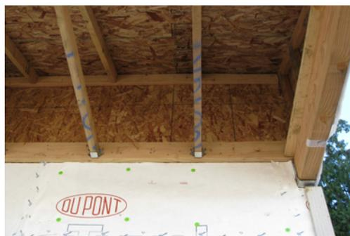
(top) Seams are caulked to provide a good air seal before installing insulation and dry wall.
