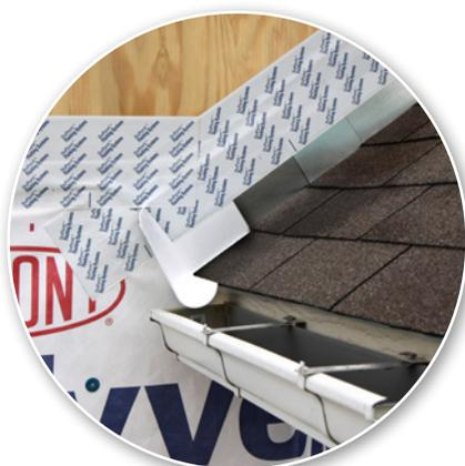
**STEP 5** Apply self-adhesive flashing over top of wall flashing, diverter, and housewrap.
