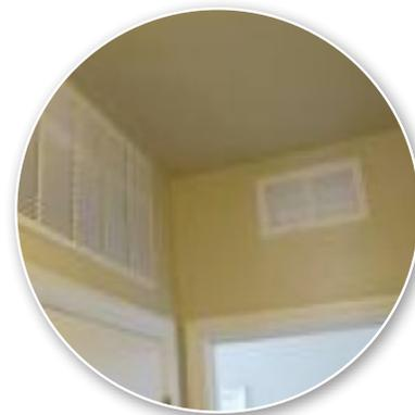
*Air handler is located in the home in a closet with return grill above. Transoms over interior doors provide a return air path.*
