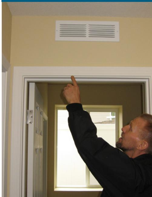
(left) Installing jump ducts from room to room is one way to balance pressures. (Photo source: IBACOS)
