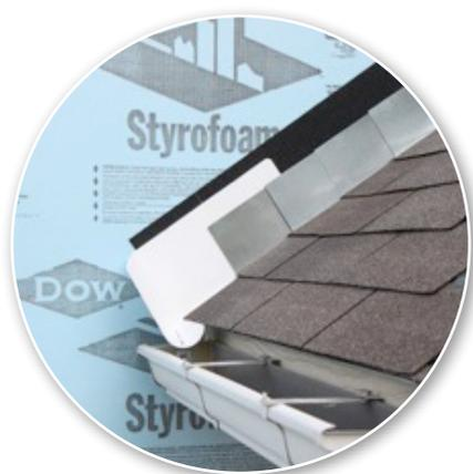
**STEP 4** Install remaining sidewall flashing, appropriate counter flashing and shingles in accordance with manufacturer's instructions.
