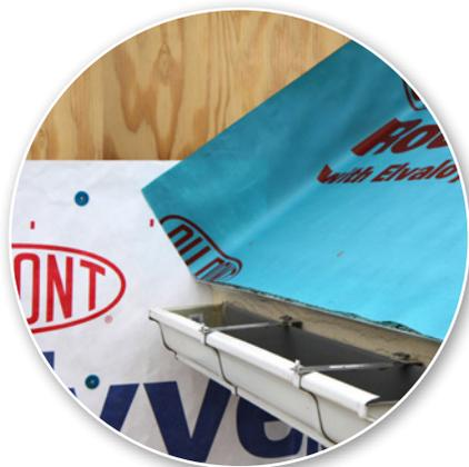
**STEP 1** Apply drip edge and roof underlayment over roof deck. Continue lapping up the sidewall and over the water-resistant barrier (in this case housewrap) a minimum of 6 inches.
