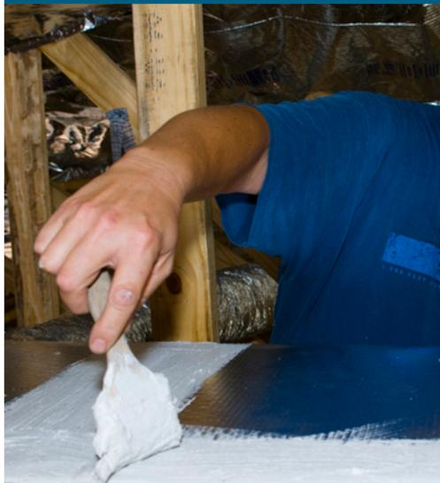
(Bottom) Mastic provides the most reliable duct sealing method. Ducts should be located in conditioned space.
