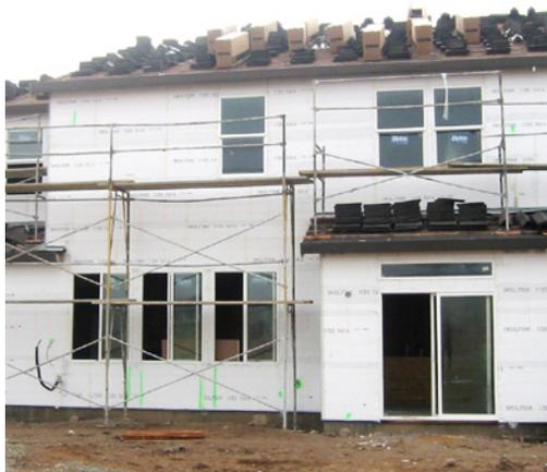
Taped rigid foam insulation can serve as a drainage plane, air barrier, and vapor barrier as well as a thermal boundary behind a stucco cladding. If using housewrap instead, never apply stucco directly to plastic housewrap. Provide a drainage space to prevent wetting of the housewrap or use two layers of textured building paper.
