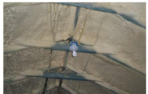
(1) Batt insulation in ceiling. (2) Blown-in insulation. (3) Spray foam. (4) Spray foam applied along the underside of the roof deck to provide a conditioned and non-vented attic space for ducts and air handlers.
