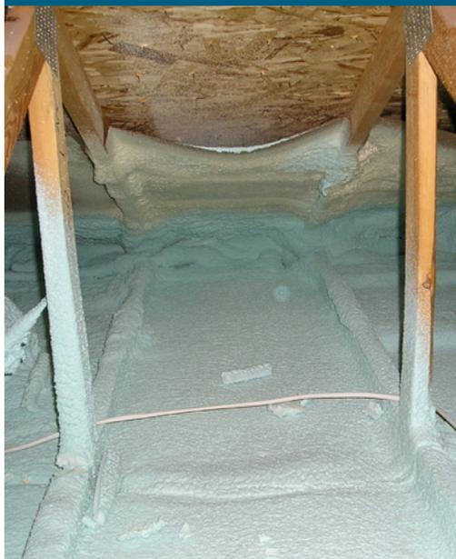
(left) Spray foam is used to insulate and air seal the “lid” or ceiling deck and any ducts located in the attic in Devoted Builders’ homes in Pasco, Washington. The spray foam is covered with more than 12 inches of blown cellulose for the equivalent of R-49 of attic insulation.
