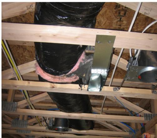
(Top and Bottom) These Building America builders run ducts through open-web floor trusses to keep the ducts in conditioned space (shown here). Open-web trusses allow subcontractors the flexibility to run plumbing, electrical, and ductwork easily between floors, with little to no “trade damage” or “trade fighting.” Air handlers are located in conditioned space in the home or in an air-sealed closet in the garage.
