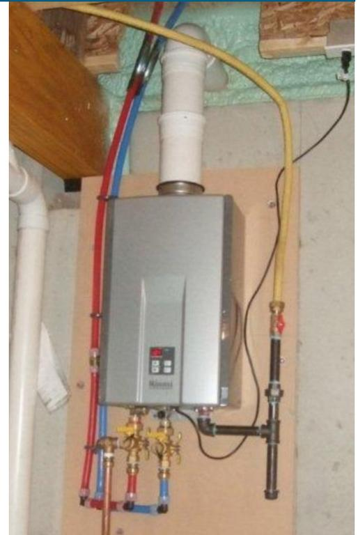
The tankless gas-fired water heaters installed by Nelson Construction in Farmington, Connecticut, save energy by eliminating the stand-by losses inherent with storage tank water heaters.
