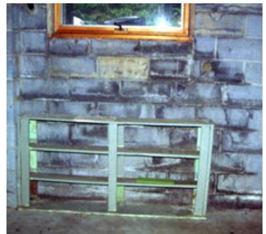
(top) When moisture is trapped inside walls, mold can grow unchecked, causing damage to the walls and health impacts for the occupants. (Photo source: EPA; photo by Terry Brennan)
