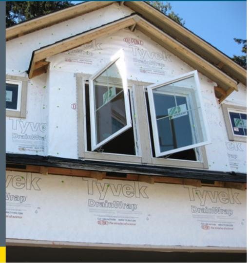
In its simplest form, building envelopes are cubes that incorporate three parts: the floor, four walls, and a roof. In actuality, these assemblies are complicated combinations of rectangles, triangles, and even domes. Building homes that deliver comfort, durability, and energy performance requires paying attention to the details of each assembly. This chapter provides guidance on controlling liquid and water vapor, air flow, and heat flow in the foundation, wall, and roof assemblies.
