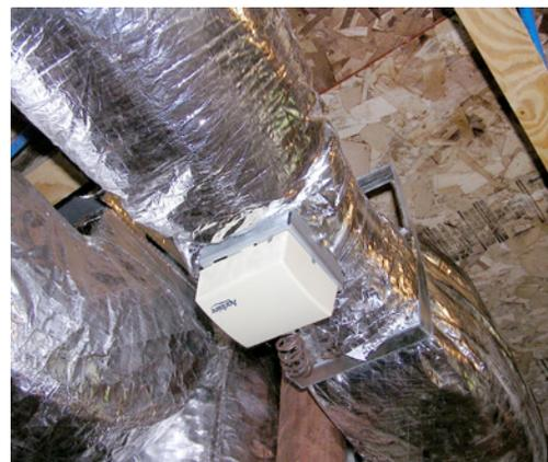
Nelson Construction attached a fresh air intake with a timed mechanical damper controller to regulate fresh air flow into the return plenum of the HVAC air handler. The damper can be set to open allowing fresh air to be pulled into the air handler by the air handler fan, also operated by the timer. This draws fresh air into the house at regular intervals. When combined with timed exhaust fans, this provides low-cost balanced ventilation.
