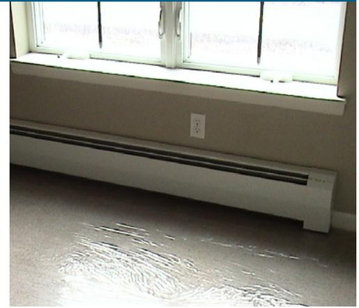
Hydronic heating in condominiums in Aspen, Colorado, uses water that is preheated by solar thermal panels, then heated by a gas boiler, and distributed via baseboard radiators.
