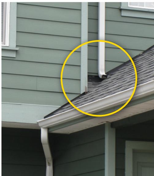
Water should not be directed to flow into the wall. This could soon lead to water intrusion in the wall.
