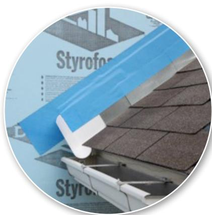
**STEP 5** Apply self adhesive flashing over top of wall flashing, diverter and rigid foam insulation.
