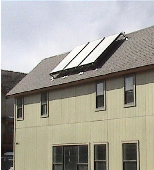
Solar water heating panels were mounted on each multifamily building to provide domestic hot water and pre-heat water for the hydronic baseboard space heating system.
