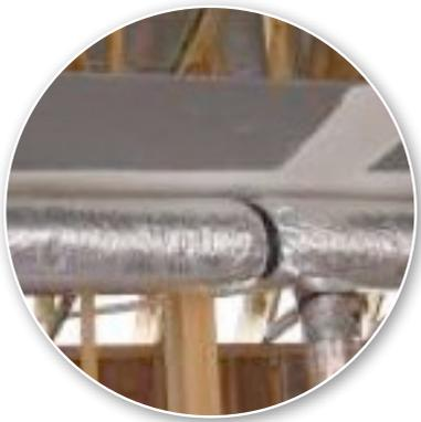
**STEP 7** Install sheetrock around ducts to form chase, when sheetrocking the rest of the house (this is the second visit for sheetrockers).
