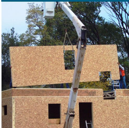
Builder David Sullivan and the South Chicago Workforce worked with Building America on the first structural insulated panel (SIP) home project ever permitted in the City of Chicago. SIPs provide excellent air sealing and insulating properties with fewer seams to caulk and much less thermal bridging than typical stud construction.
