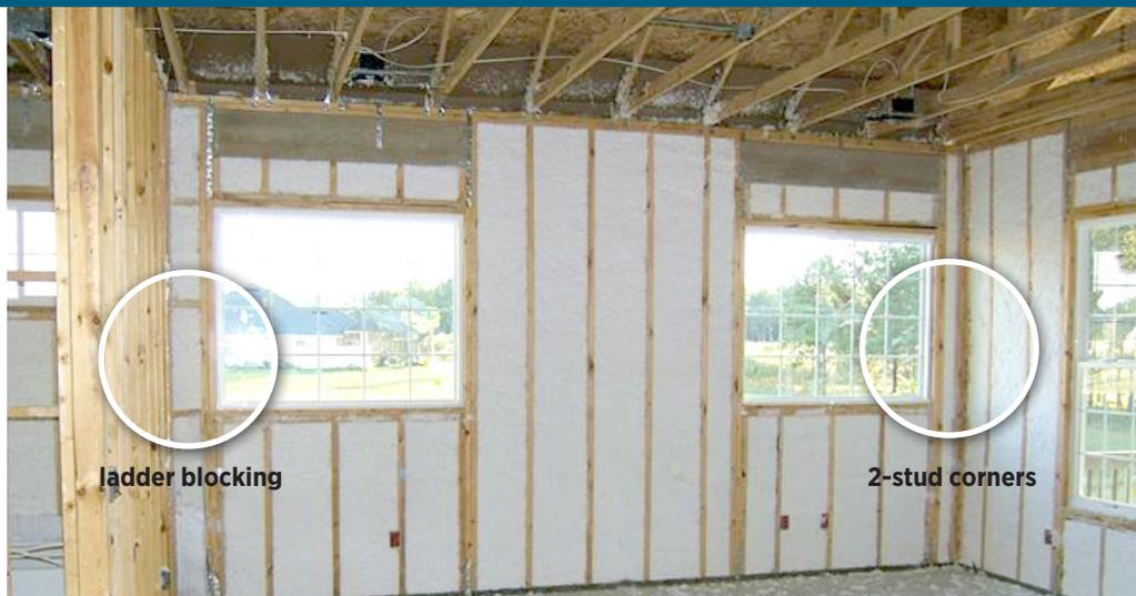
(left) Sheet goods come in 4x8-foot dimensions. Designing and building on a 2-foot grid saves cutting time and reduces lumber and sheet good waste.
