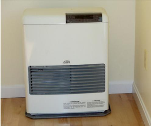
The homes are so well insulated that a 10,200-Btu gas-fired space heater on the main floor, (shown in wood cabinet in top photo and alone in bottom photo), provides all the heat needed.
