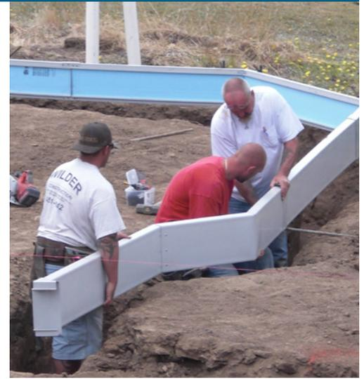
Davis Energy Group of the CARB Building America team developed a method for insulating slab perimeters. The method, which is commercially available, uses termiticide-treated rigid foam insulation encased in PVC as the form for the concrete foundation. In cold climate locations, the forms can be stacked to provide deeper protection against frost (Personal communication with David Springer, Davis Energy Group, 11/10/10).
