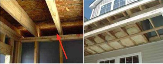
Left: This cantilevered floor (viewed from the inside) does not yet have air sealing or insulation installed. (Photo source: Energy Services Group).
