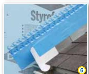
Installing Sidewall and Kick-out Diverter Flashing
