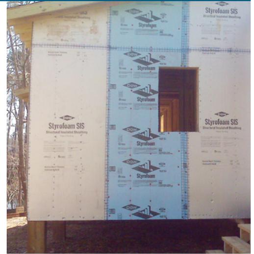
**Exterior rigid foam.** Rigid foam insulation is installed on the exterior of a new framed home in Georgia. The rigid foam takes the place of OSB wall sheathing (Photo Source: IBACOS).
