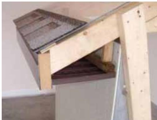
The fascia was redesigned to extend 1 inch below the soffit to form a drip edge, directing water down and away from the house.
