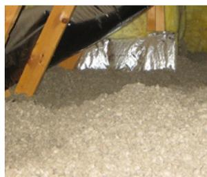
Loose fiberglass insulation
