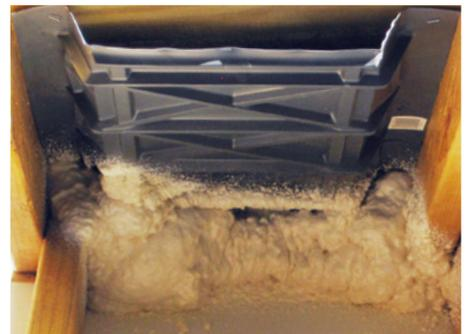
**Figure 5.5. Baffles.** Your contractor will install vent baffles to maintain a 2-inch continuous ventilation channel above the insulation.
