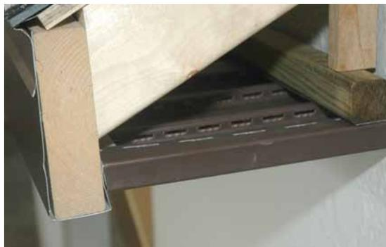
Perforated soffit board product with recessed openings was installed to limit water intrusion while encouraging greater air circulation and faster drying within the eave assembly.
