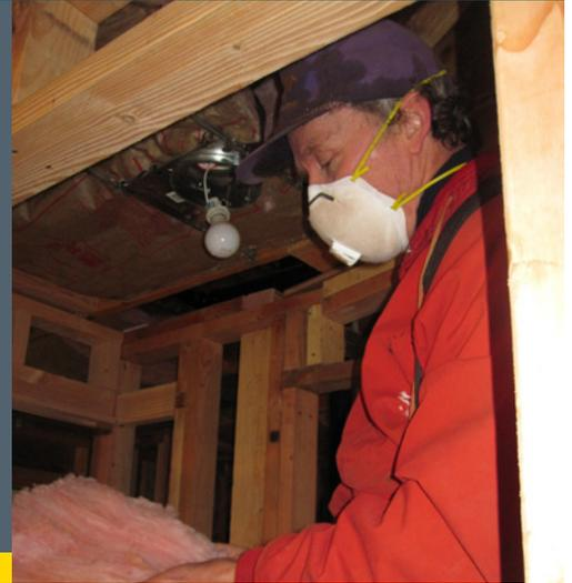
Your home may not be well insulated. The insulation may be too thin, uneven, or missing altogether. Cracks, leaks, or vents in walls, floors, ceilings, or roofs may allow air to flow through your insulation, reducing its effectiveness. Adding insulation and sealing air leaks can make your home more comfortable, increase its value, and cut your utility bills.
