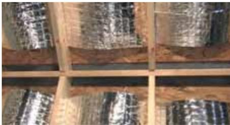
In hot climates, radiant barriers can cut cooling costs 8% to 12%. In this house, a flexible radiant barrier material was draped over the rafters before installation of the roof deck. The material also can be stapled to rafters from the underside (Photo Source: Universal Forest Products).
