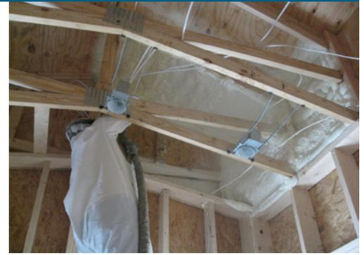
**Polyurethane foam insulation.** Leave the installation of spray foam to trained professionals. Toxic gases emitted during application are hazardous to skin, eyes, and lungs (Photo Source: NAHB).
