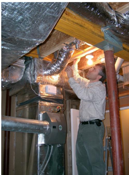
*(Top)* Mastic is a thick, gooey substance that is painted onto seams and joints. Duct seams and joints should be sealed with mastic or approved metal tape, not duct tape (Photo Source: FSEC).
