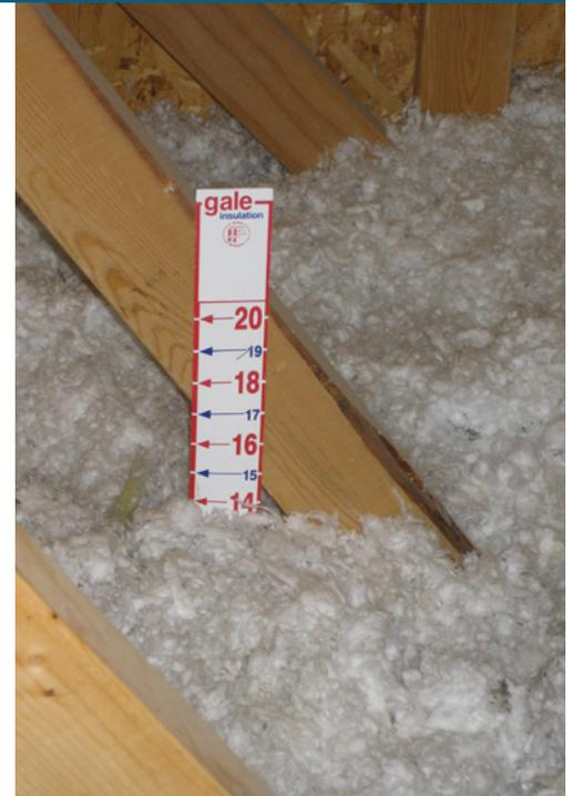
**Depth of insulation.** When installing loose-fill insulation in an attic, your contractor should staple rulers in several places to ensure the insulation is deep enough and has been spread evenly. These rulers are also useful for measuring changes over time as insulation settles (Photo Source: PNNL).
