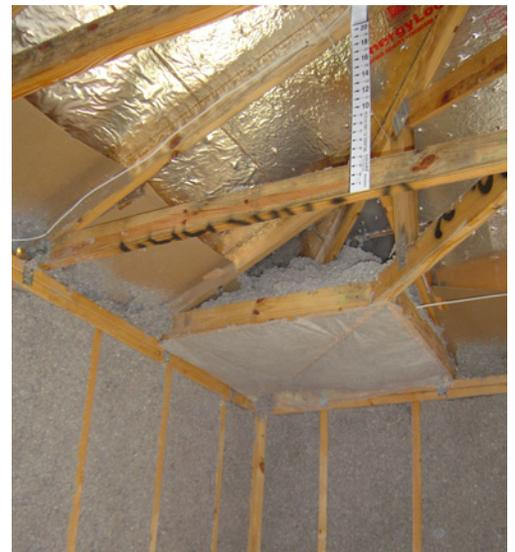
(Top) **Dense-pack fiberglass.** In this newly built home, dense-pack fiberglass is held in place with netting. This is a popular choice for retrofit insulation, blown into open cavities or installed using the drill-and-fill method (Photo Source: Bob Ward Company).
