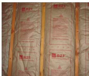
Faced fiberglass batt insulation
