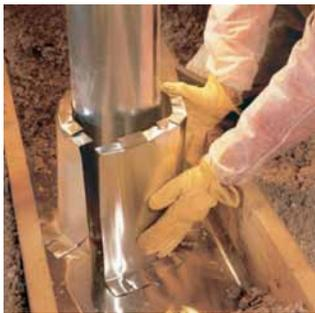
You can make a sheet metal or gypsum board dam to keep insulation from touching hot metal or masonry chimneys and flues (Source: EPA 2008a).
