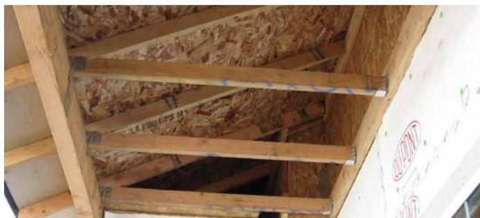
When the wall connecting the porch to the house is properly blocked and air sealed with OSB, dry wall, or rigid foam, a significant source of air and heat loss is removed.
