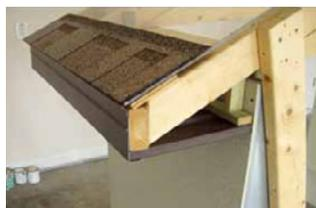
Typical soffits have a fascia that is level with the bottom of the vent panel and vent perforations that face downward allowing rain water dripping down the fascia to be blown or drawn into the vent openings.
