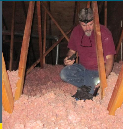
Insulation is made of a variety of materials that have a high thermal resistance, which means resistance to heat flow. The unit of measure for a material's thermal resistance is its R-value. The R-value of insulation depends on the type of material, its thickness, and its density. The higher the R-value, the greater its insulating effectiveness.
