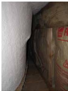
This tub was installed without a proper air barrier, such as cement backer board or rigid foam, to cover the batt insulation. The batt's paper facing doesn't form a continuous air barrier so air can flow through the wall cavity.
