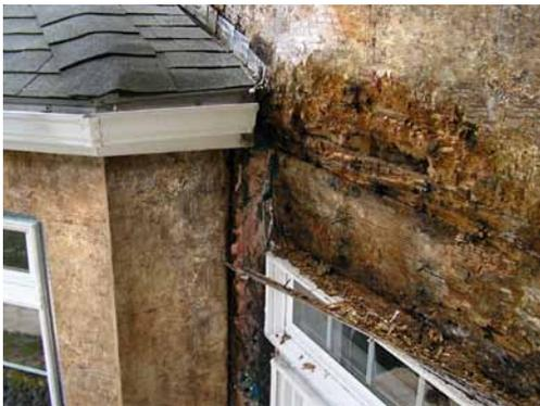
Improper flashing can allow rain water into walls, causing significant damage (Source: DryFlekt Products, Inc).
