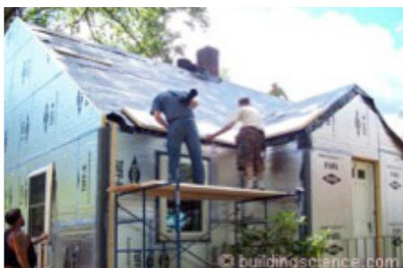
**Exterior insulation.** Workers installed a continuous air barrier on the above-grade portions of the house, including the roof, then wrapped it again with continuous layers of insulation.
