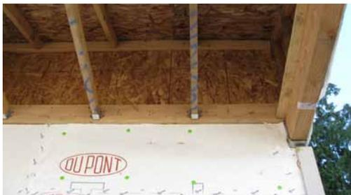
The house wall separating the porch attic from the rest of the house was correctly air sealed in this new home to prevent air from flowing into the home and causing heat loss.
