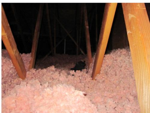
**Fiberglass.** Take care when handling fiberglass insulation, which can irritate skin and lungs. Keep kraft facing on batts away from hot fixtures. Install vent baffles to keep loose-fill insulation from blocking attic vents. Blocked vents can lead to problems with moisture, mold, and wood rot (Photo Source: PNNL).
