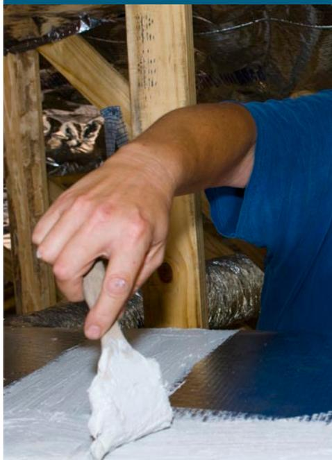
Figure 11.1. Paint mastic (a thick, goeey substance) on to the duct seams and joints. (Photo source: Habitat for Humanity Lakeland FL).
