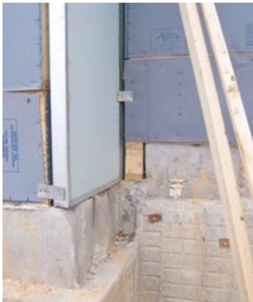
Figure 19.1. Seal air gaps between two framed common walls (Source: Energy Services Group, from EPA 2008)
