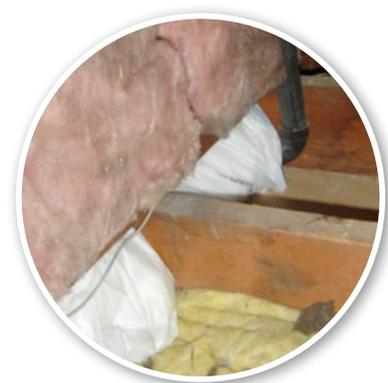
Figure 3.2. Air seal floor joist cavities under kneewalls by filling cavities with fiberglass batts that are rolled and stuffed in plastic bags (as shown here) or use rigid foam, OSB, or other air barrier board cut to fit and sealed at edges with caulk.
