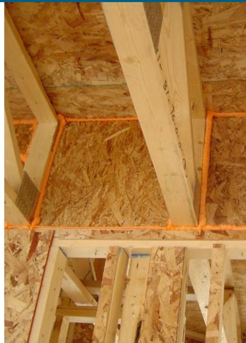
15.2. Seal rim joists of the wall separating the house's living space from the garage with pieces of wall board and spray foam.
