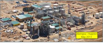
Abengoa Bioenergy Biomass of Kansas, LLC, is in the process of designing and constructing a biorefinery facility to produce cellulosic ethanol in Hugoton, Kansas. The process utilizes an enzymatic hydrolysis process to produce ethanol, process steam, and all electrical power required to operate the facility via an integrated biorefinery and cogeneration system. Initial feedstocks that will be used are corn stover and wheat straw, with other
