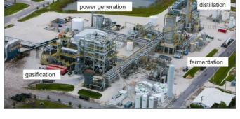
INP BioEnergy has completed construction and commissioning and is now starting operations of the first commercial-scale facility employing the INEOS Bio bioenergy process technology on a site in Indian River County Florida (known as the Indian River BioEnergy Center). The facility will produce eight million gallons per year (mgpy) of cellulosic ethanol and 6 megawatts (gross) of electricity at full rates. The project is demon-
