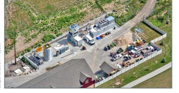
The Waste-to-Energy Cogeneration Project at Centennial Park has allowed methane from the closed Centennial landfill to completely power the recreational facility and export excess power into the grid for resale. This project is part of a greater brownfield reclamation project to the benefit of the residents of Munster and the general
