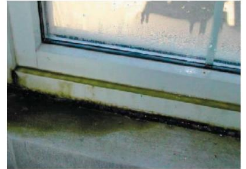
Condensation damage to wall surround (Building Envelope Forum) – S O'Brien
