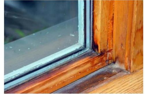
Moisture and damage to a wood window sash and frame
