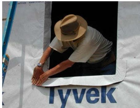
Installing window flashing. *Photo courtesy The Building America Solution Center Image Gallery.*
