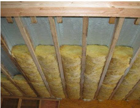
Spray foam air seal and insulation.
