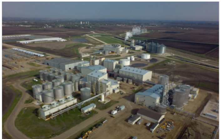
An aerial shot of POET-DSM's Project LIBERTY cellulosic ethanol plant in Emmetsburg, Iowa. Photo courtesy of POET-DSM
